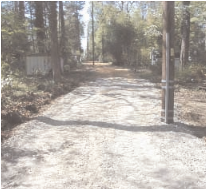
Construction loads will now be properly supported with a geotextile-reinforced road.
