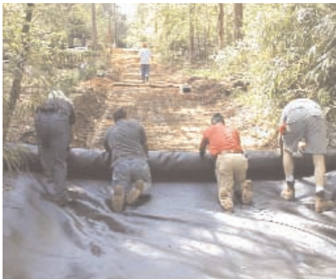
Mirafi® HP370 is installed after the road is graded.
