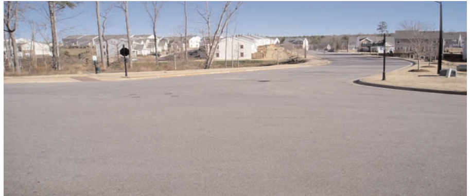
HP reinforced intersection at Country Trail and Marvino Lane.
