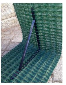
The internal braces are designed to integrate with PYRAMAT 75 HPTRM and provide internal structure during construction to facilitate placing and backfilling of PYRAWALL. The bracing members are designed to interlace through PYRAMAT 75 HPTRM resulting in superior material connection and system performance throughout the project's design life.
