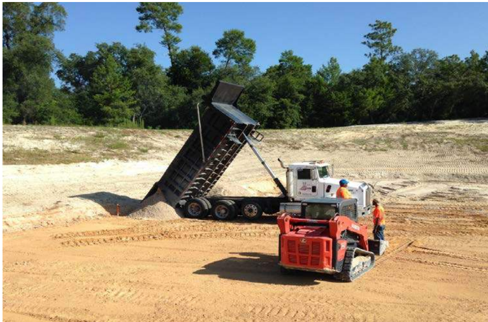
Figure 10 Installation of the BAM in the one-acre RIB
