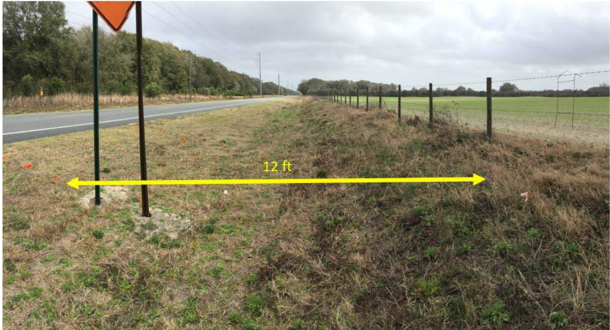
Figure 35. Linear ditch construction site
