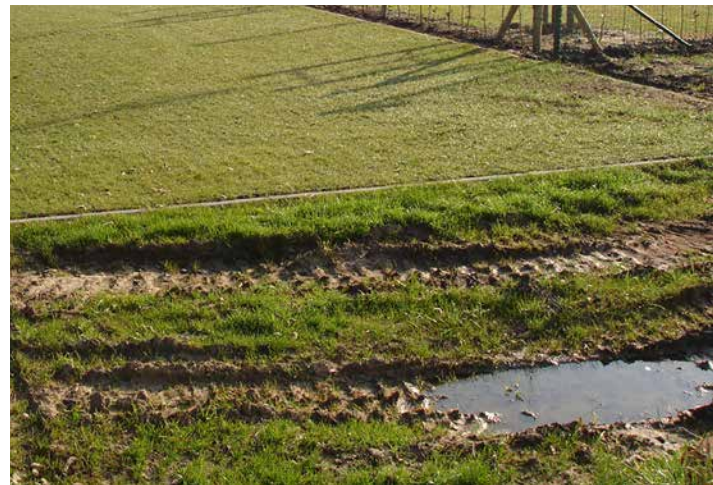
E-40 Permeable Surface vs. Unsupported Surface
