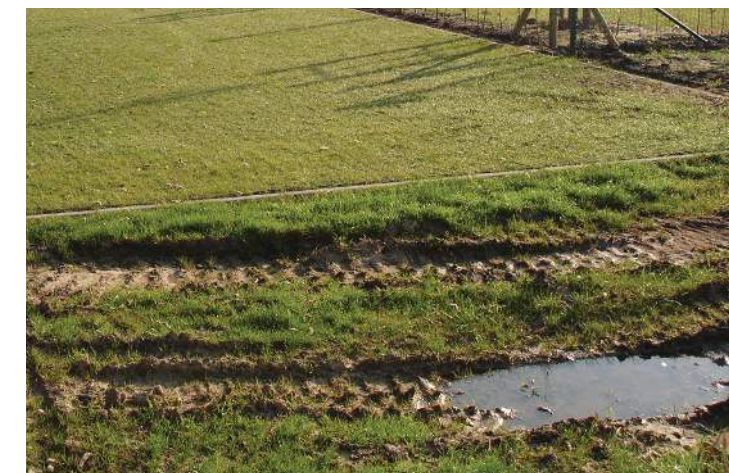
E-40 Permeable Surface vs. Unsupported Surface
