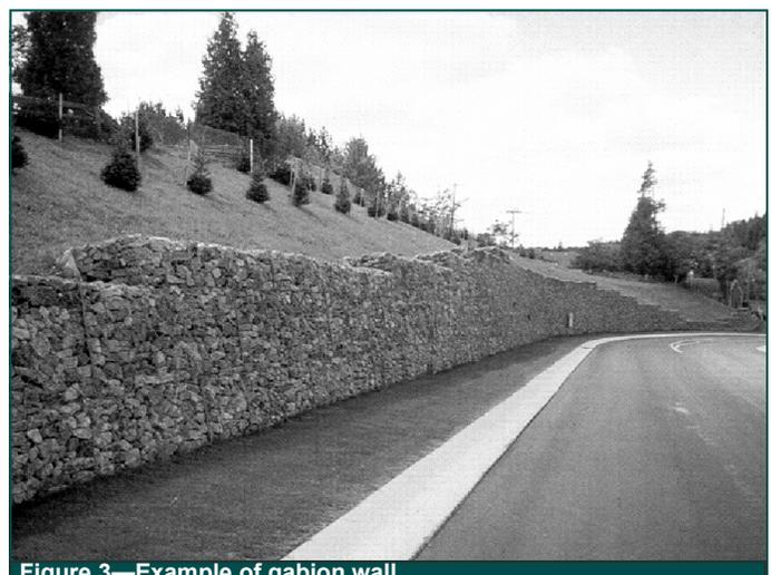
Figure 3—Example of gabion wall
