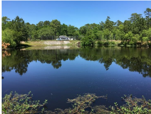
Figure 5. Wilmington Operations Center wet pond.
