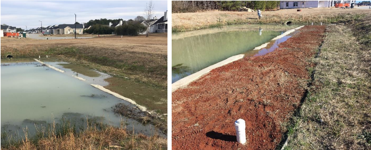
Figure 16. Biological blinding of the shelf filter observed at the Sapphire pond (left) remedied by raking of the filter surface (right).
