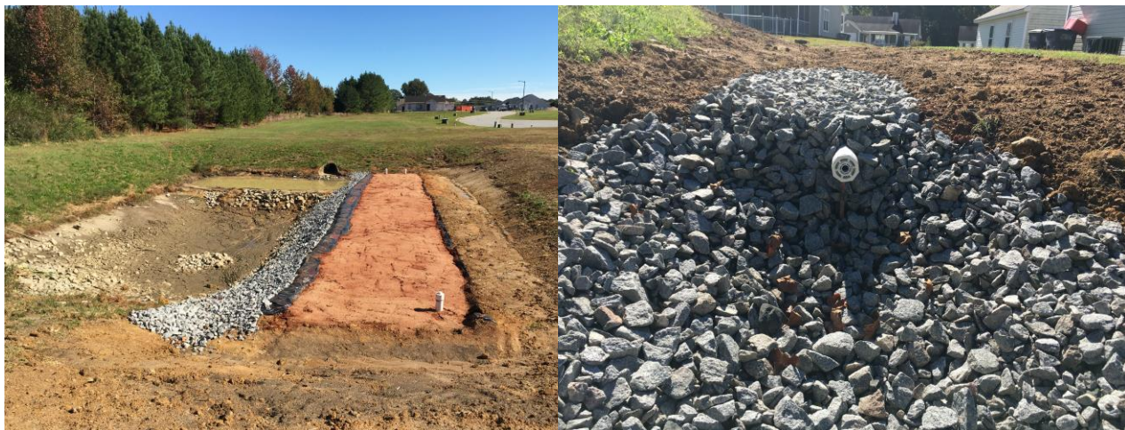
Figure 2. Sapphire littoral shelf filter following construction (left) and underdrain (right).
