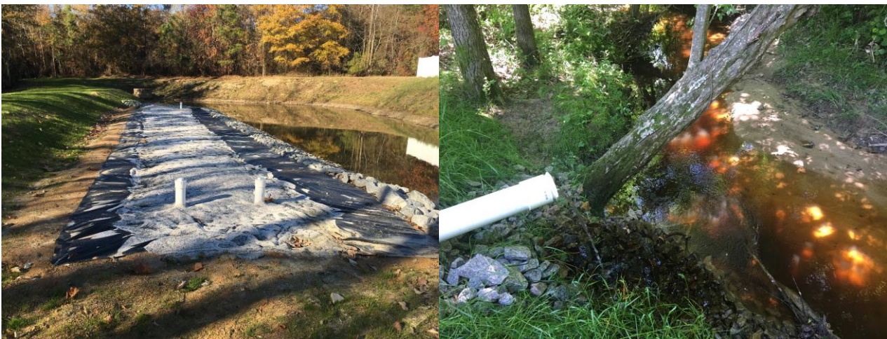
Figure 4. Bridgewood littoral shelf filter following construction (left) and underdrain (right).
