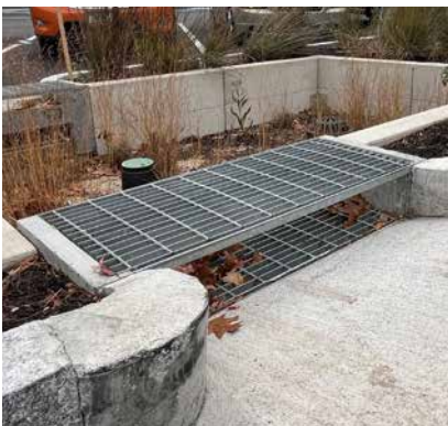
Highly urbanized bioretention
