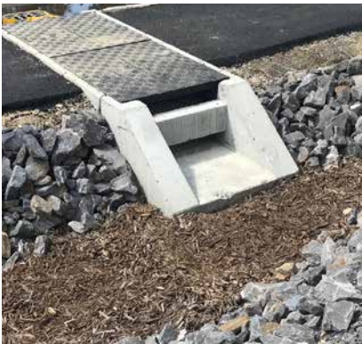
Routing runoff under paths and boulevards
