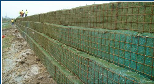
TenCate Miramesh® geogrids provide some of the highest UV durability reinforcement available, allowing for permanent green face walls and slopes.
