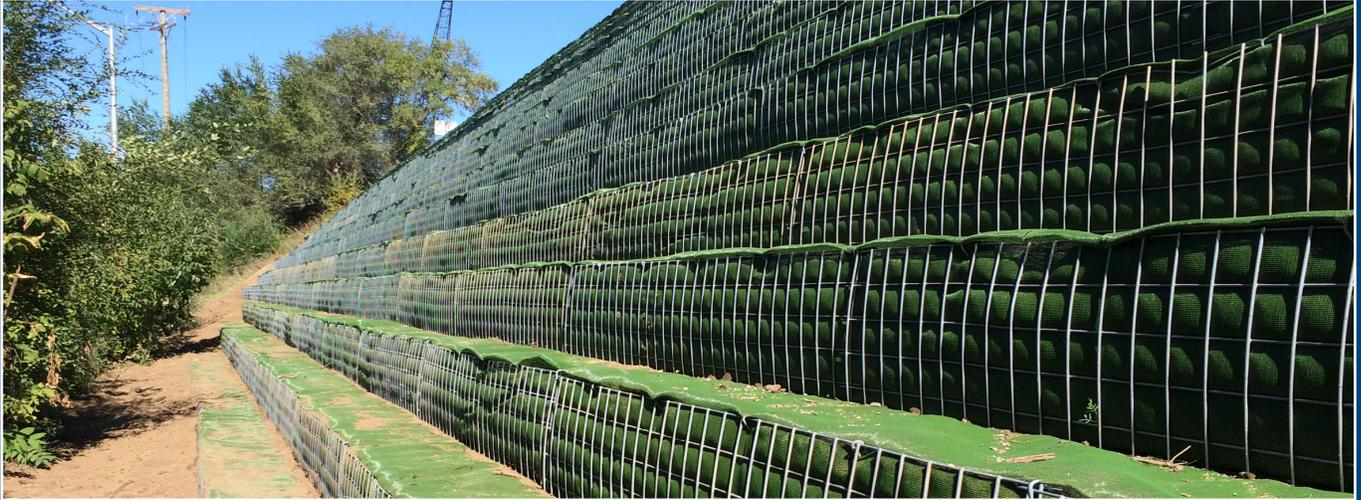
Cherry Island Landfill is one of the largest vertical expansion berms in North America, measuring over 65' tall and almost a mile long. The reinforced berm utilizes high-strength geotextile material with a tensile strength of over 80,000 lb/ft.
