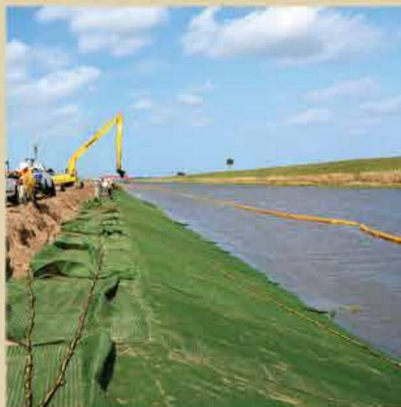
Woven TRMs can be deployed to provide a range of performance and durability options: Medium Loading/Survivability | High Loading/Survivability | Anchor Reinforced Vegetated System
