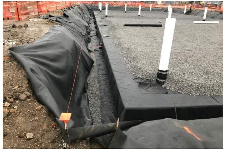
Side backfill and geotextile wrap.
