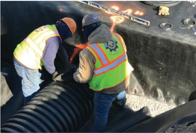
Connection of pipes with geotextile boot kits.
