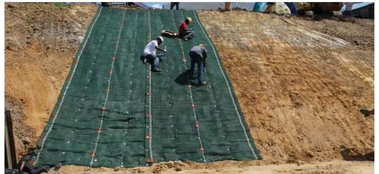
Beginning of Armormax install with Pyramat rolled down the hill and washer pins installed.
