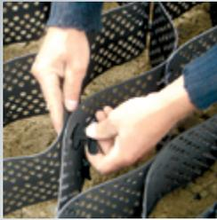
For quick and easy connection of GEOWEB® sections, exclusive ATRA keys significantly reduce contractor installation time and provide a 3X stronger connection of GEOWEB® sections than any other method. Made from corrosion-resistant polymer.
