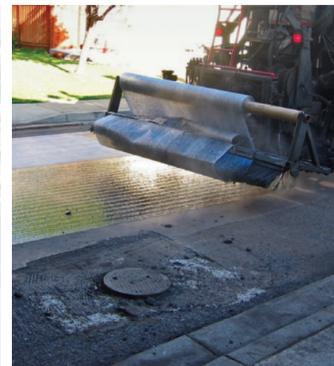
With proper design and placement, interlayers can add traffic capacity to the asphalt pavement.
