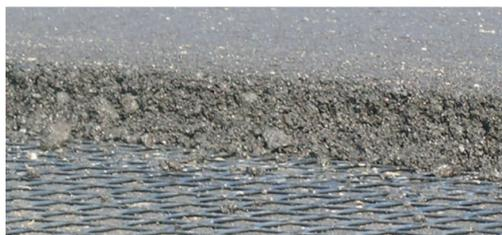
GlasGrid Pavement Reinforcement System
