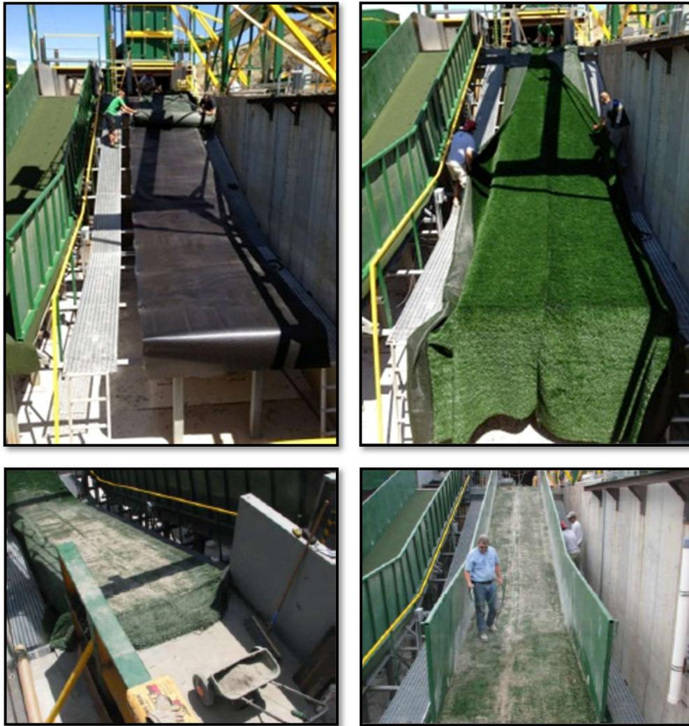
**Figure 3. HydroTurf® System Installation**
