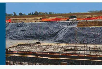
PVC (Polyvinyl Chloride) geomembranes were developed for applications such as landfills, canals, ponds and other containment purposes. They are formulated to withstand atmospheric pollutants and chemicals commonly found in industrial settings.
