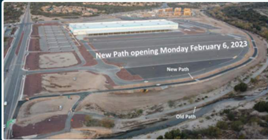
Silverbell Gateway Distribution Center, Amazon
